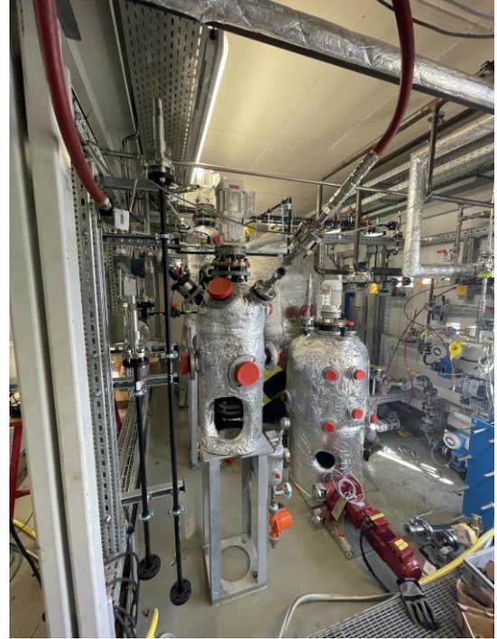
Figure 5 The Inlet Brine Cooling system
