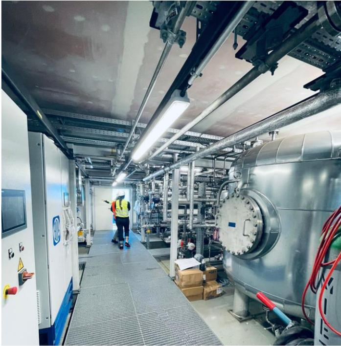
Figure 4 Water Storage tank from Water preparation system
